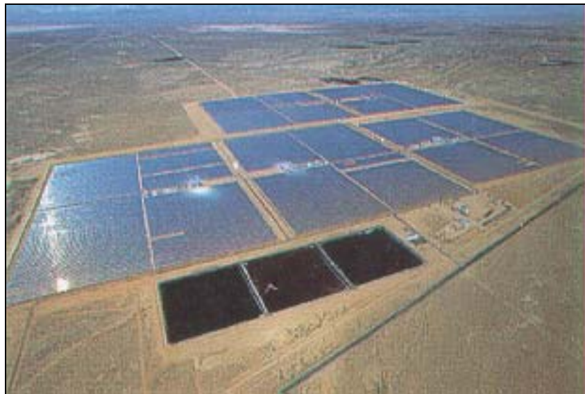
Figure 1: 5 x 30 MW electric SEGS plant at Kramer Junction, California (Source: Flachglas Solartechnik GmbH, Köln).
